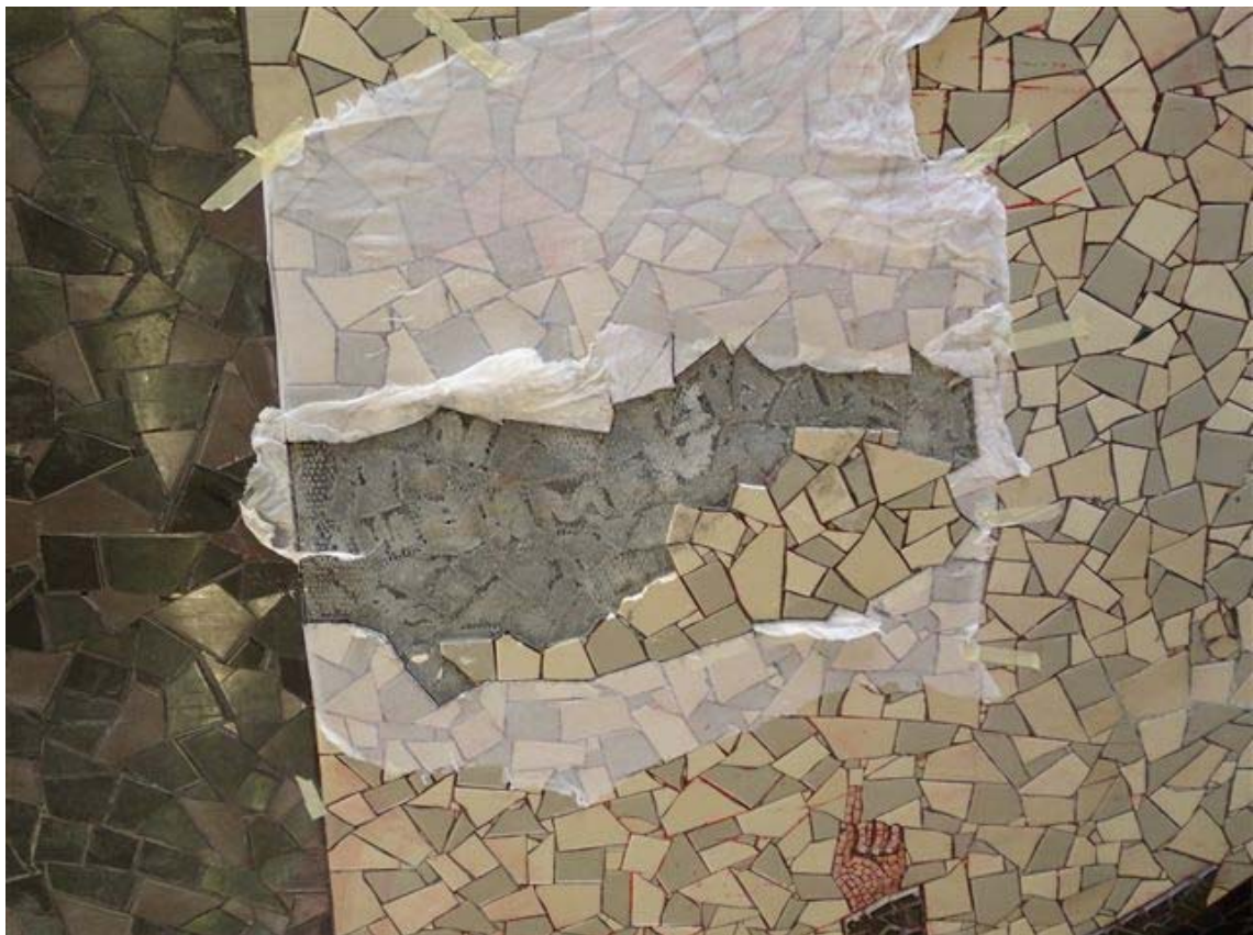
Trial area with tiles removed from brick facing leaving E.M.L. attached
