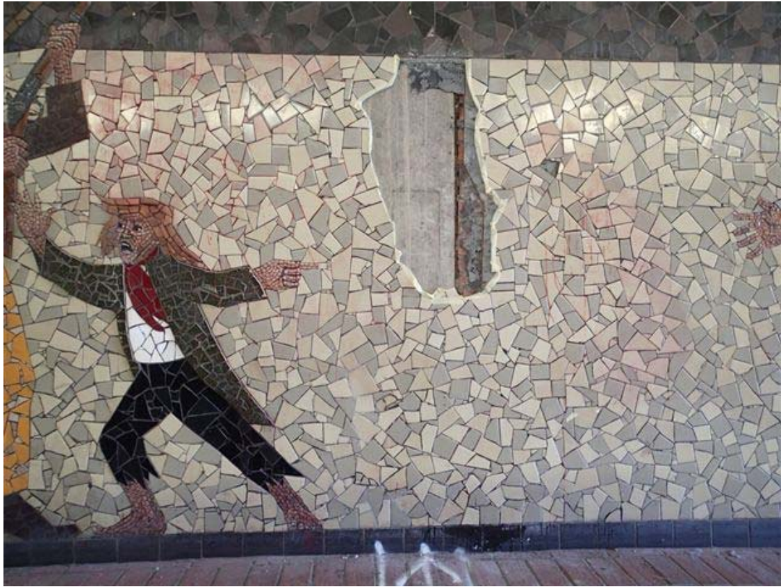
Trial area section removed from concrete pier
