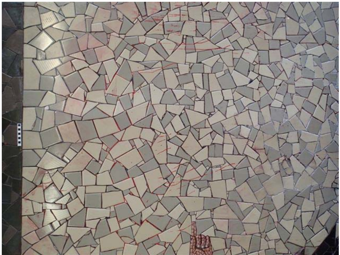
Trial area before commencement of work
