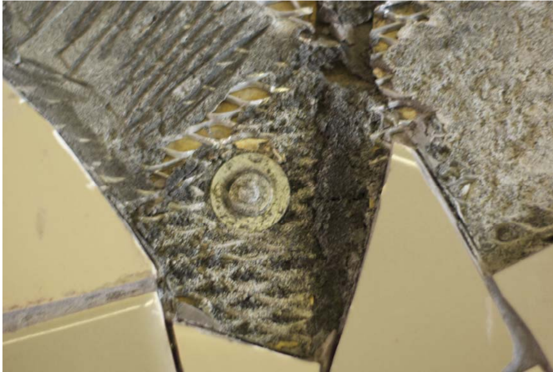
Example of 'Hilti' fixing of E.M.L. to brickwork
